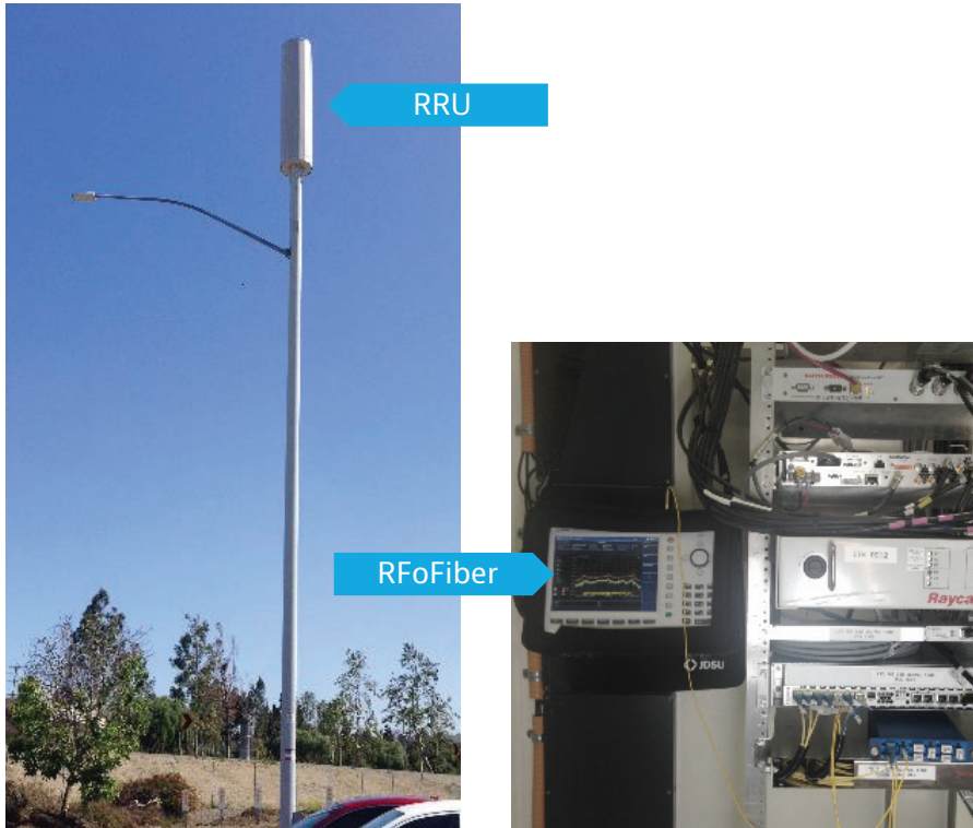
Figure 9. Small cell and CellAdvisor with RfFiber
